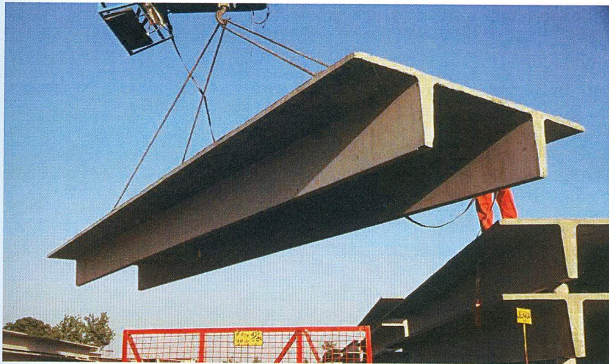
Double Tee Plant in Lahore
