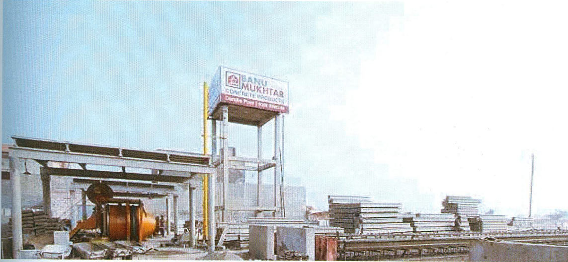
Pre-Cast slabs Plant in Gujranwala
