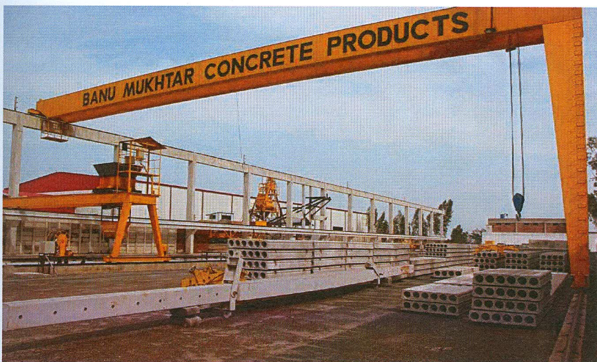
Hollow Core Plant
