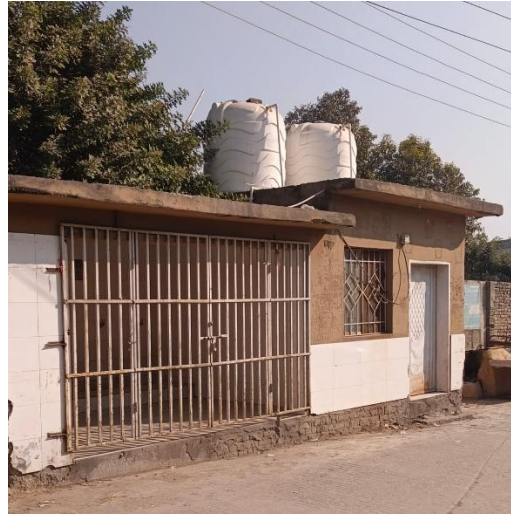
Figure No. 4.2: Community Water Filtration Plant
