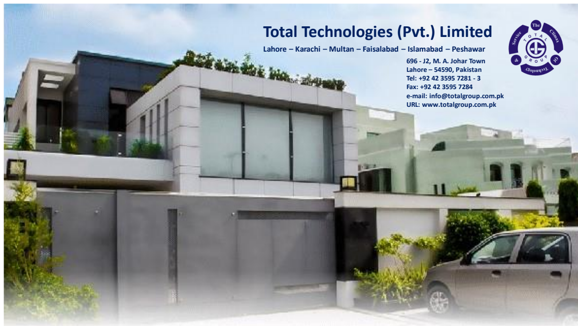
Figure 1 Total Technologies Office
