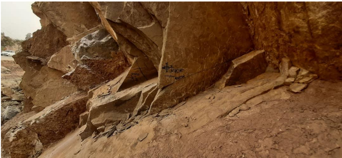
Figure 2.2 Field photographs showing conjugate joints in the sandstone within Murree Formation.
