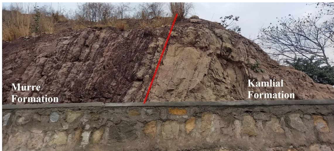
Figure 2.3 Field photography showing Contact of Kamlial Formation with Murree Formation along Islamabad Expressway near Korang bridge.
