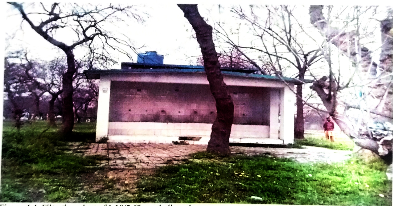
Figure 4.4. Filtration plant of I-10/2 Chanmbali road
