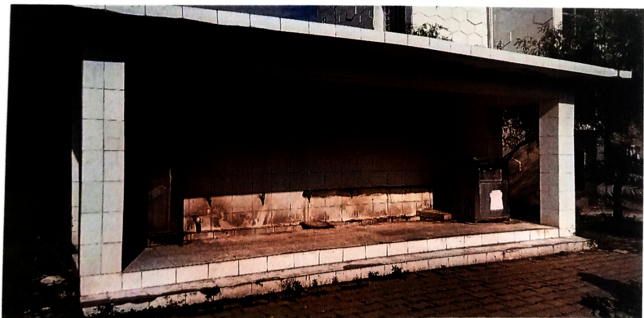
Figure 4.2. Filtration plant of Pak Secretariat P-block
