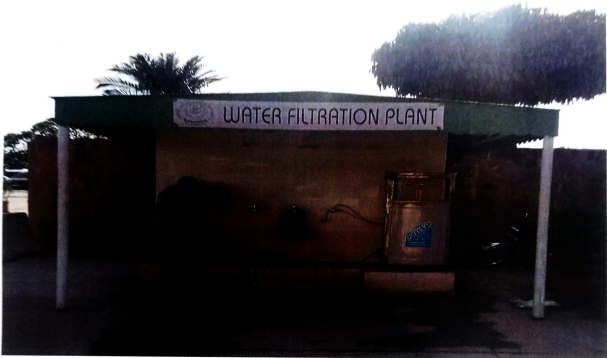
Figure 4.1. Filtration plant of Parliament house
