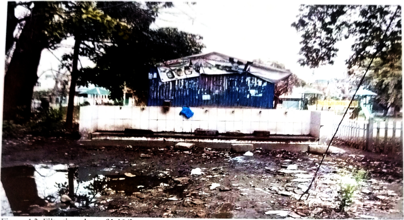
Figure 4.3. Filtration plant of I-10/2
