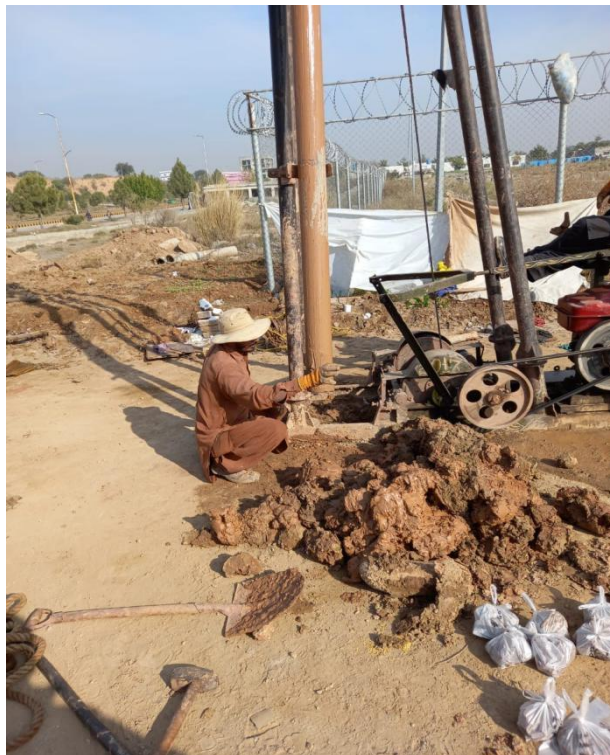
Figure 4.4. Drop hammer of 63.5kg used for SPT.
