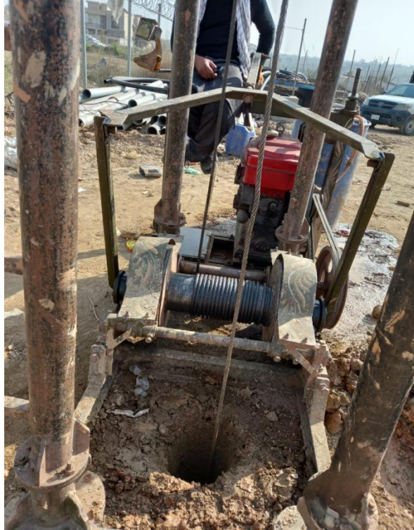
Figure 4.1. Drilling rig used for performing SPT test.
