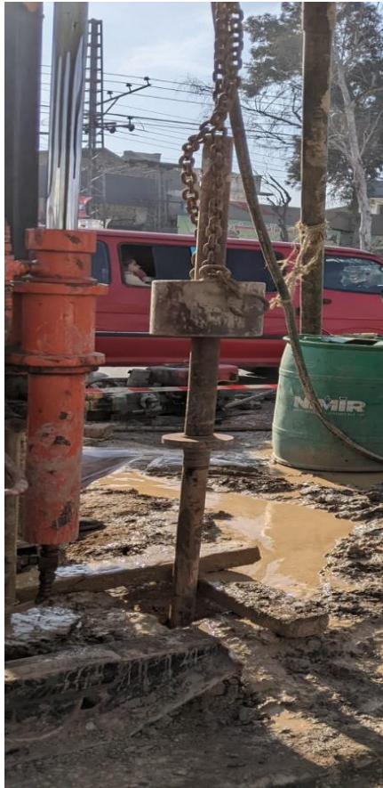
Figure 4.3. Drop hammer of 63.5kg used for SPT.
