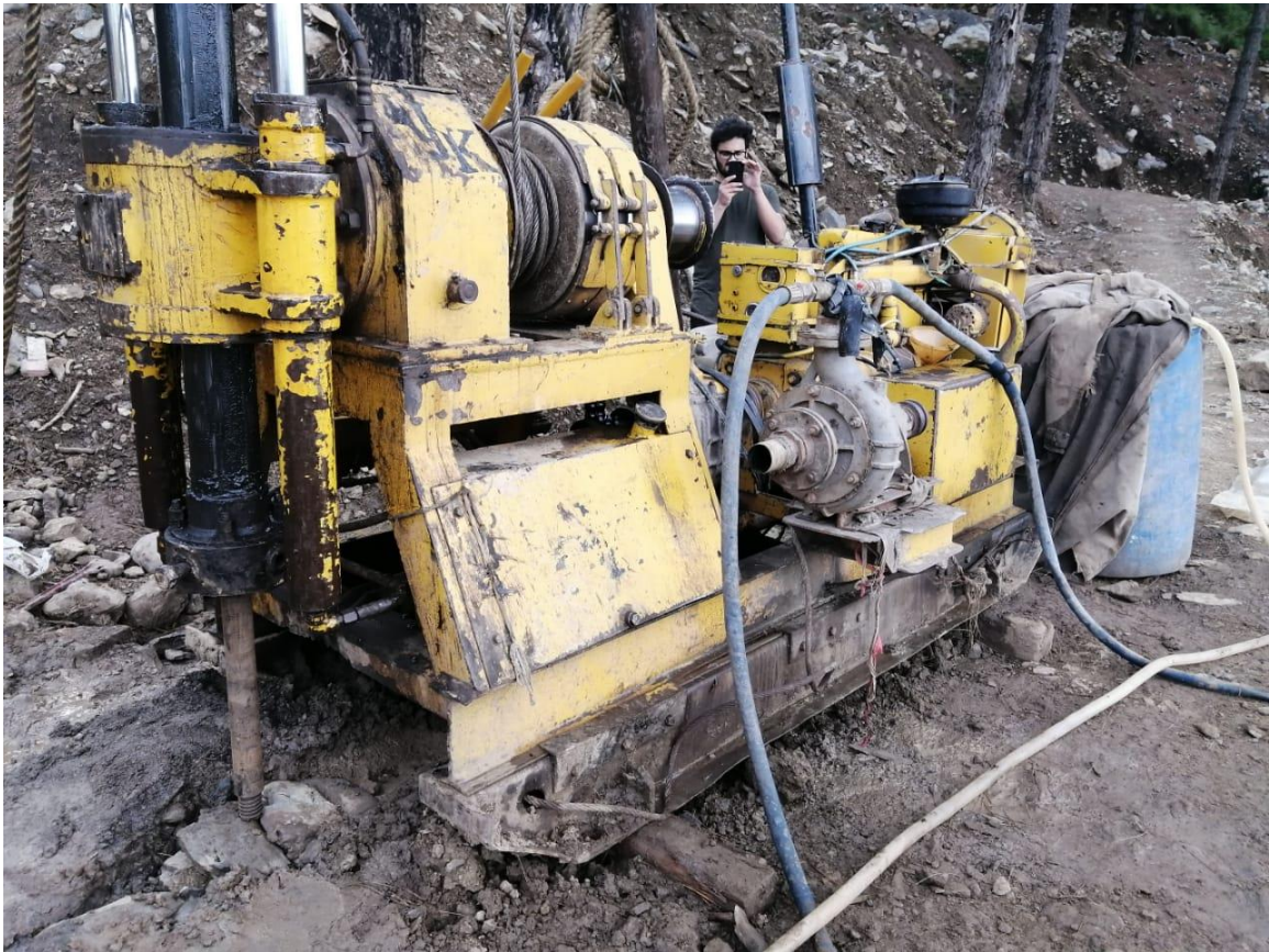
Figure 4.1. Drilling rig used for performing SPT test.
