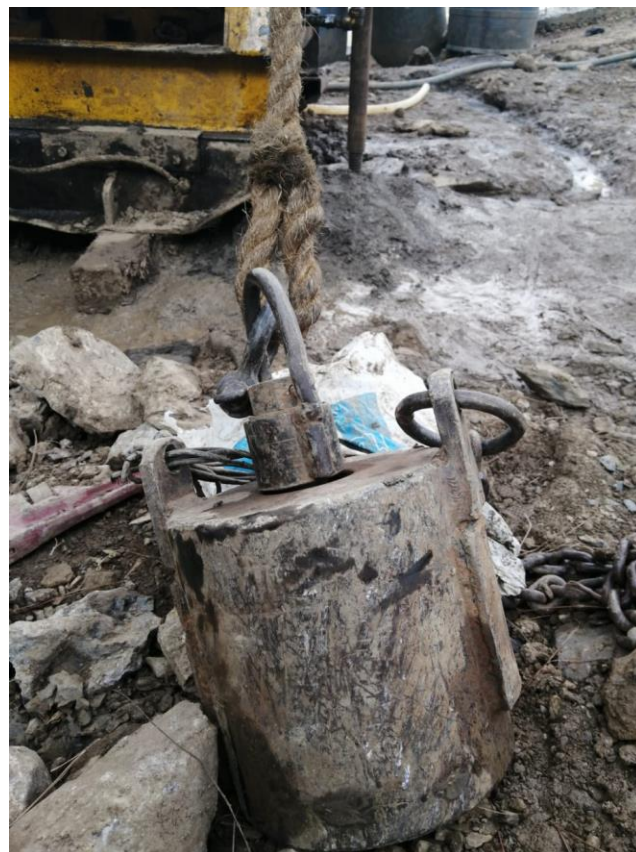
Figure 4.4. Drop hammer of 63.5kg used for SPT.
