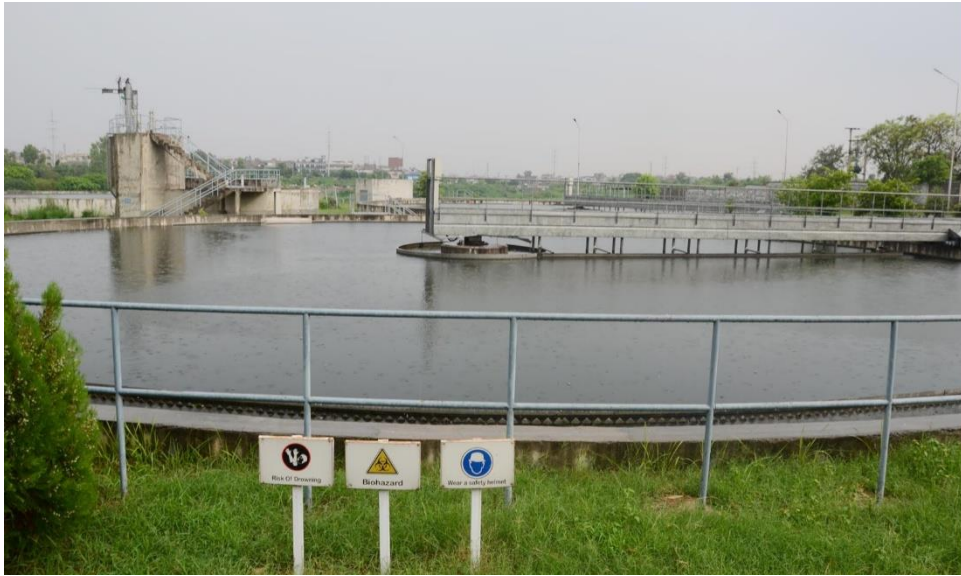
Figure 7 Islamabad I-9 Waste water treatment plant
