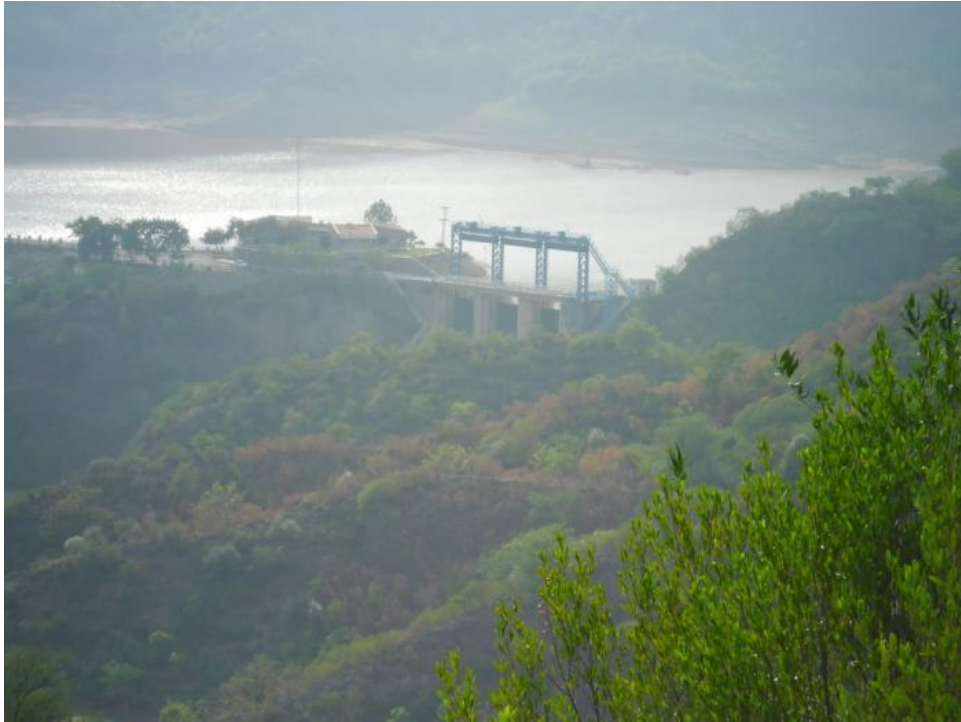
Figure 9 Simly dam raw water treatment plant
