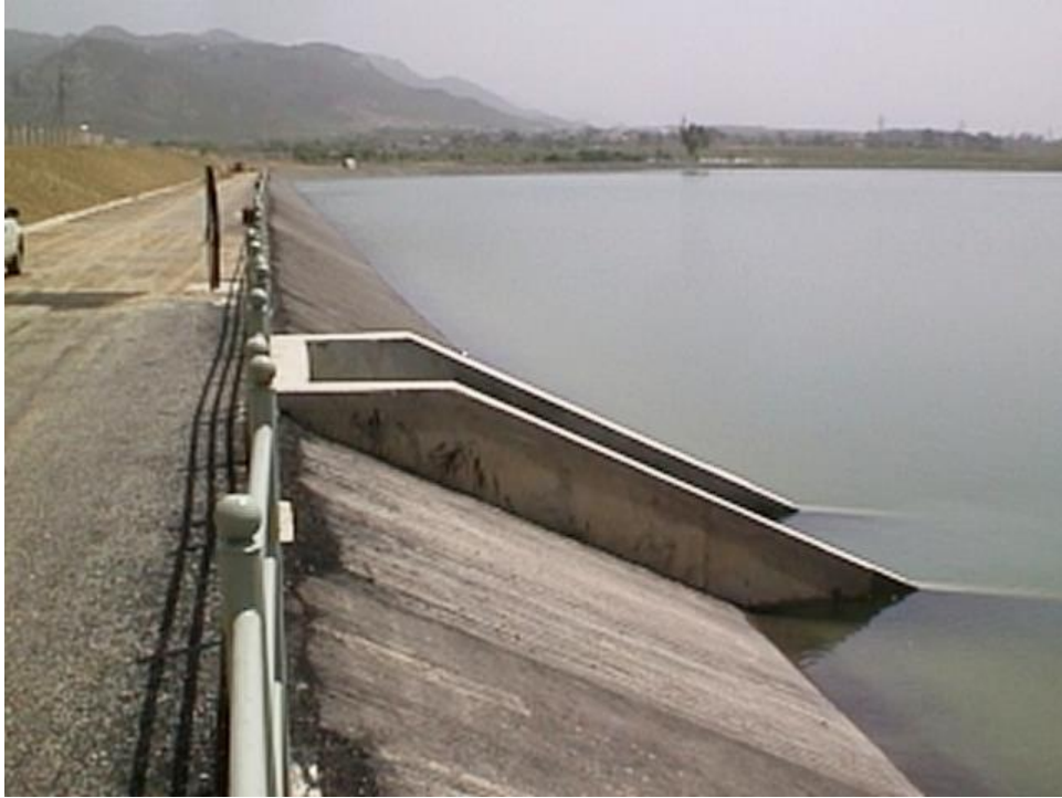
Figure 8 Khanpur dam Sinjani raw water treatment plant
