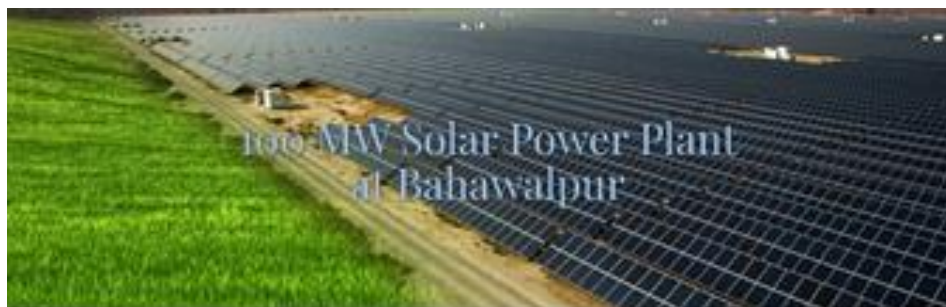
Figure 1. Quaid-e-Azam Solar Power (Pvt) Ltd
