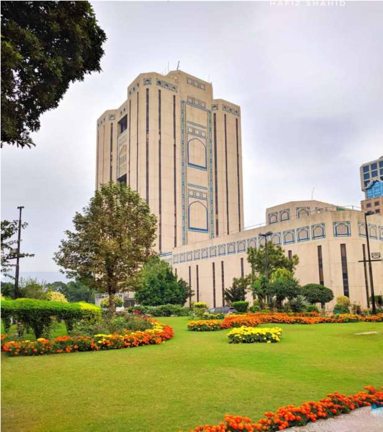
Figure 3.1 Saudi Pak Tower-Medicsi Hospital Front View F-7
