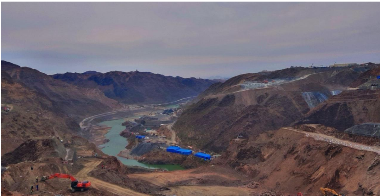
Figure 1: Construction Site of Mohmand Dam
